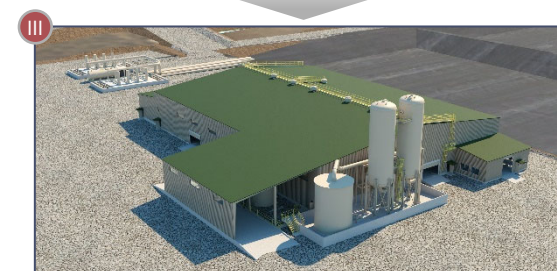
Merrill-Crowe process plant (capacity of 13,750 gpm 1 )
